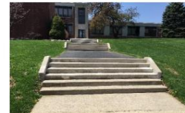
Concrete stair sections & asphalt landings/walks without railings
