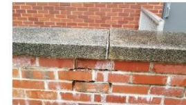
Failing brick site wall
