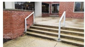
Failing site walls and stairs
