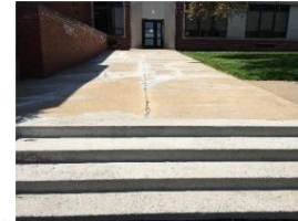
Cracked and sloped concrete walkway to bus loading area
