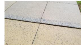
Uneven sidewalk at main entrance
